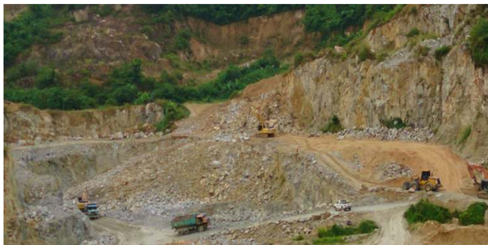
Fig. 3 View of the studied quarry
