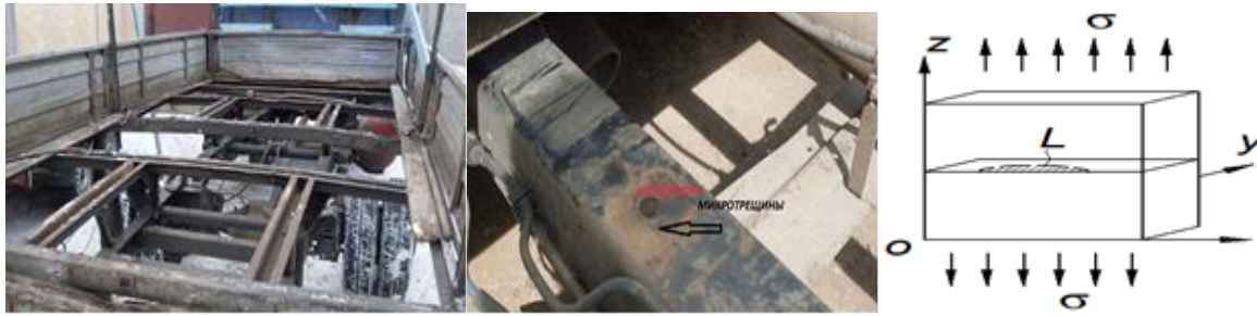
Fig. 1. Corrosion-fatigue cracks in the vehicle frame, a classical body scheme of loading a body with a flat surface crack
