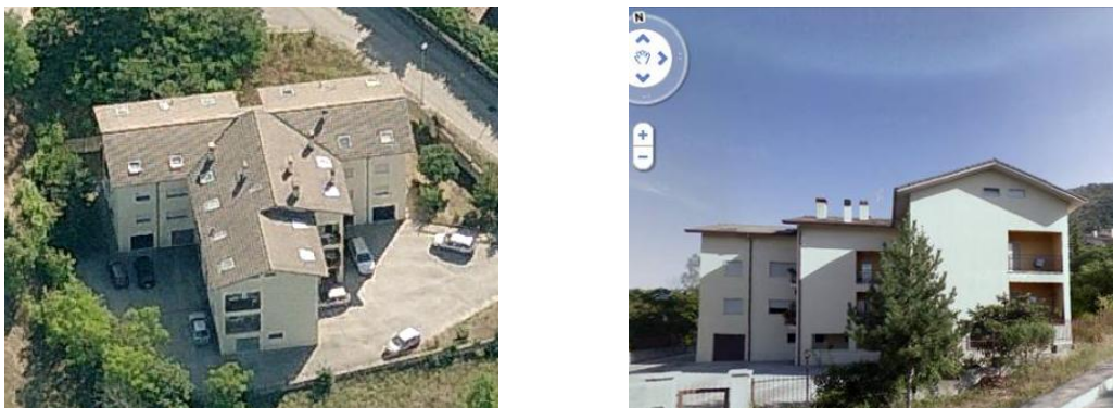
Figure 1. Pre-event view of case study building, placed in Pettino (L'Aquila) (Virtual Earth)
