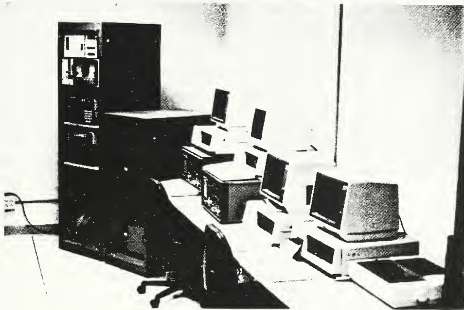
Figure 13 Photograph of Diagnostic Center Monitoring Equipment
