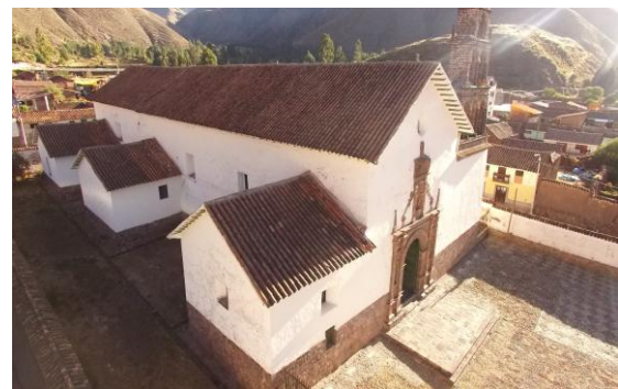
Figure 8. General view of the church.
