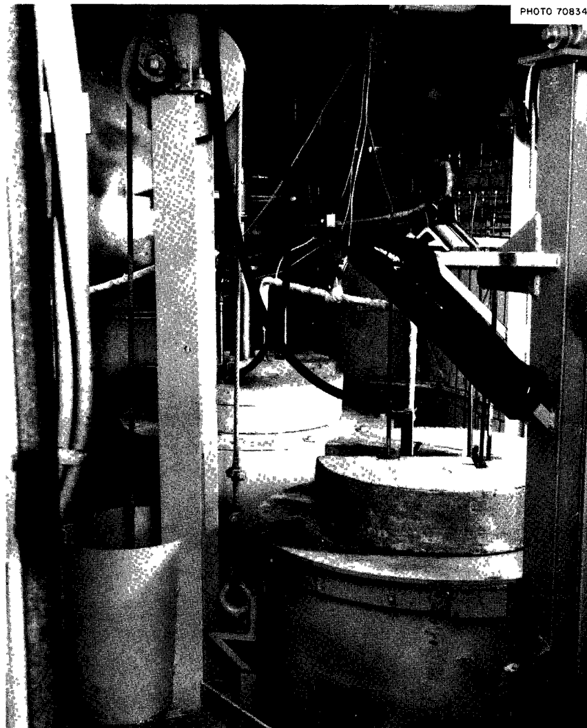
Fig. 15. Fluoride Production Facility – Batch Processing Unit.
