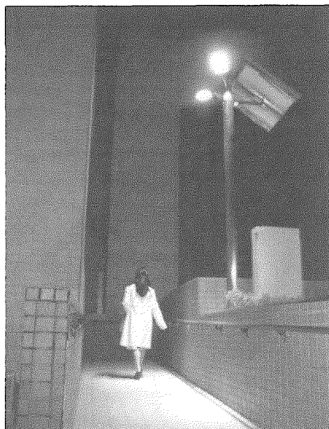
Fig. 6 White LED lighting as a street lamp in the nighttime. A maximum illuminance over 660 lx.
