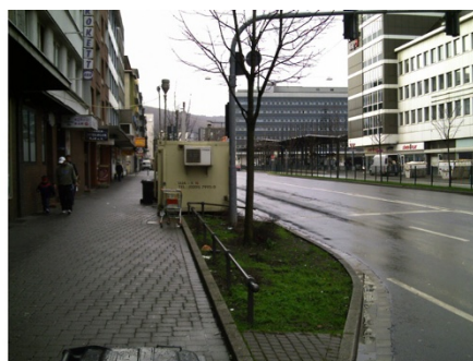
monitoring station in Hagen
