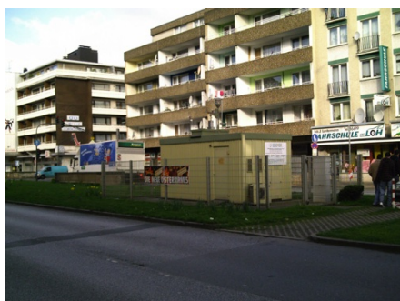
monitoring station in Wuppertal
