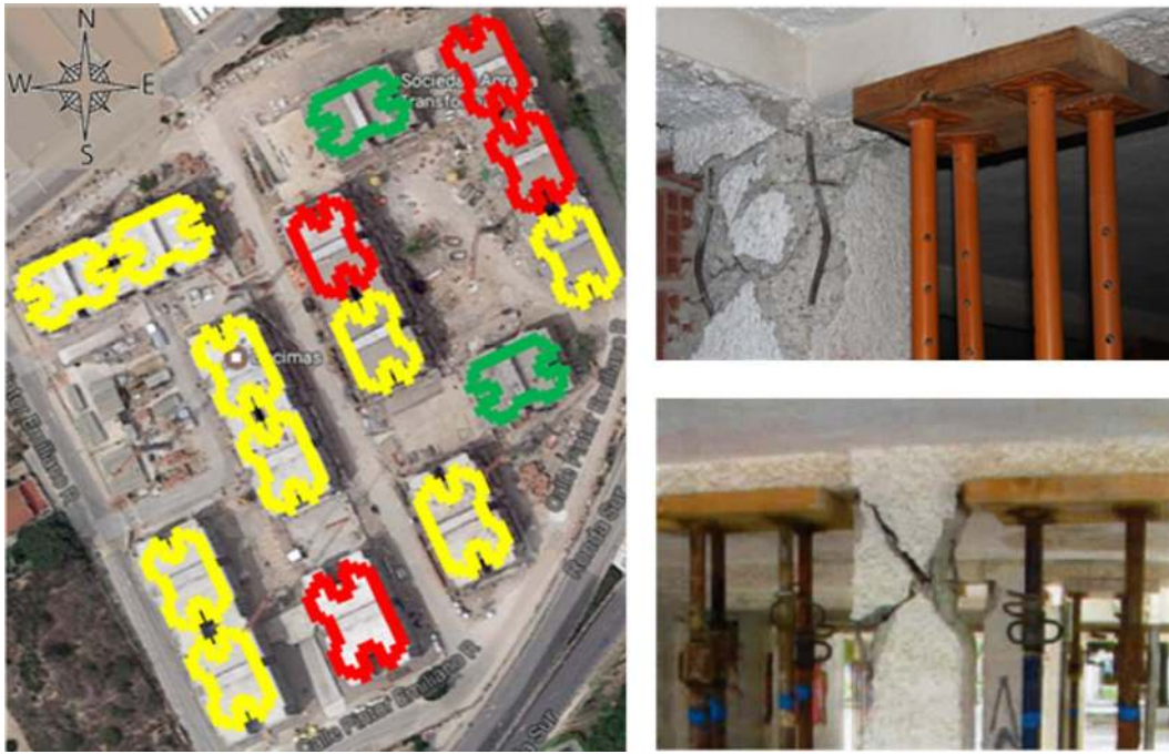
Figure 5. Plan view of the buildings located in San Fernando neighbourhood affected by the Lorca earthquake. Green colour indicates that the building was not damaged; yellow colour means that the damage is repairable and red colour indicates that the building is holding extensive damage and that there is risk of collapse.
