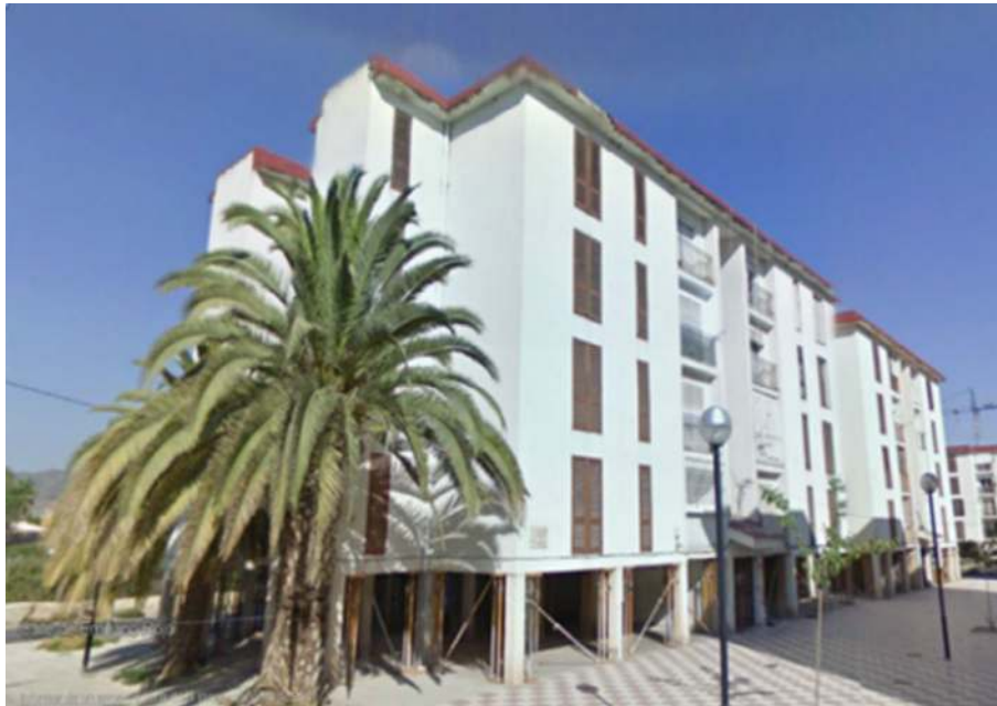
Figure 3. Buildings located in the San Fernando neighbourhood of the city of Lorca, Spain, affected by the earthquake.
