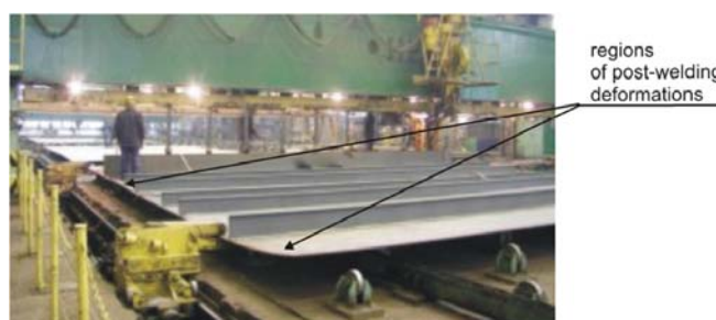
Fig. 1. Welding deformations of a plate section
