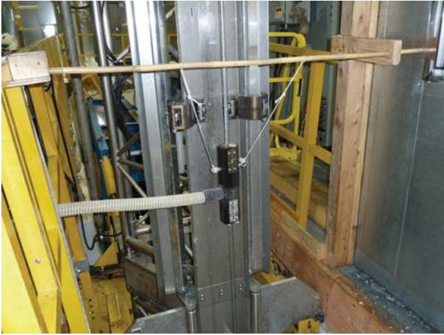
Fig. 4. Cable vacuum used during ascent of the drill.
