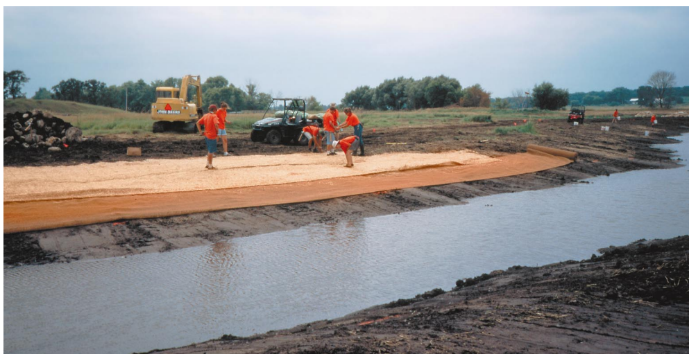
Fig. 1. A 2.6 km segment of Nippersink Creek, Illinois, USA, was filled in to make farming more efficient. Here, the meandering creek is being restored by excavating the historical channel, contouring the banks, anchoring mats to control erosion, adding a mulching blanket and seeds to encourage native vegetation, and planting propagules of aquatic plants. The project has multiple goals: reduction of flooding downstream; improved water quality; habitat for fish, wading birds and waterfowl; and involvement of youngsters in the process (Ed Collins, project director and restoration ecologist with the McHenry County Conservation District, pers. commun.). Photo by J. Zedler.
