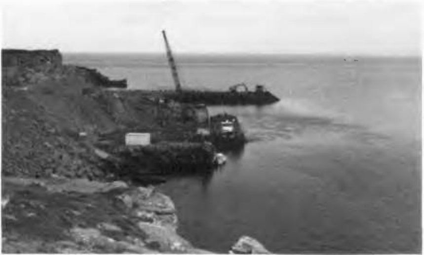
Figure 2 Quarry Operation Adjacent to Breakwater Construction
