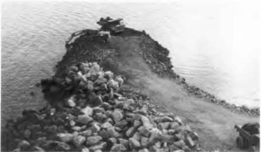
Figure 3 Breakwater Construction
