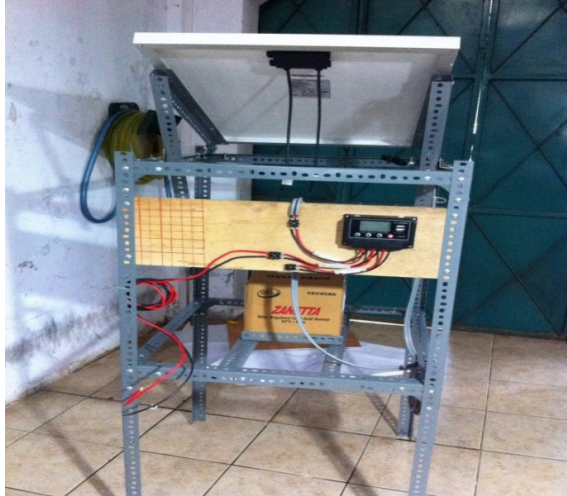
Gambar 5. Prototype Sistem Pompa Air Tenaga Surya
