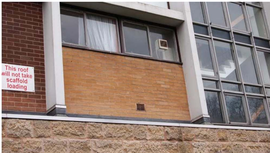
Figure 4: Close up of cladding to rear elevation.
