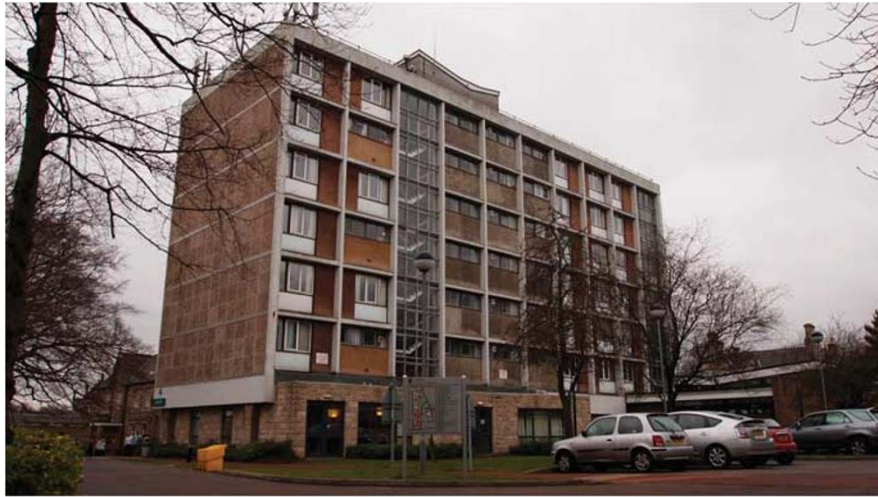
Figure 3: The building rear elevation.
