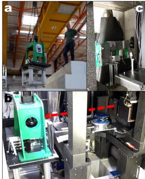
Figure 1 – PSI ‘Neutron Microscope’ at ILL-D50 beamline: (a) being installed through the open roof into the bunker, (b) positioned at the most downstream position of the ILL-D50, (c) fitted with B_4C sheets and other borated shielding materials. The red dashed arrow in Figure 2b indicates the neutron beam.
