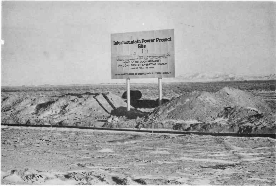
P-1. IPP Generating Station Construction Site, December 1981
