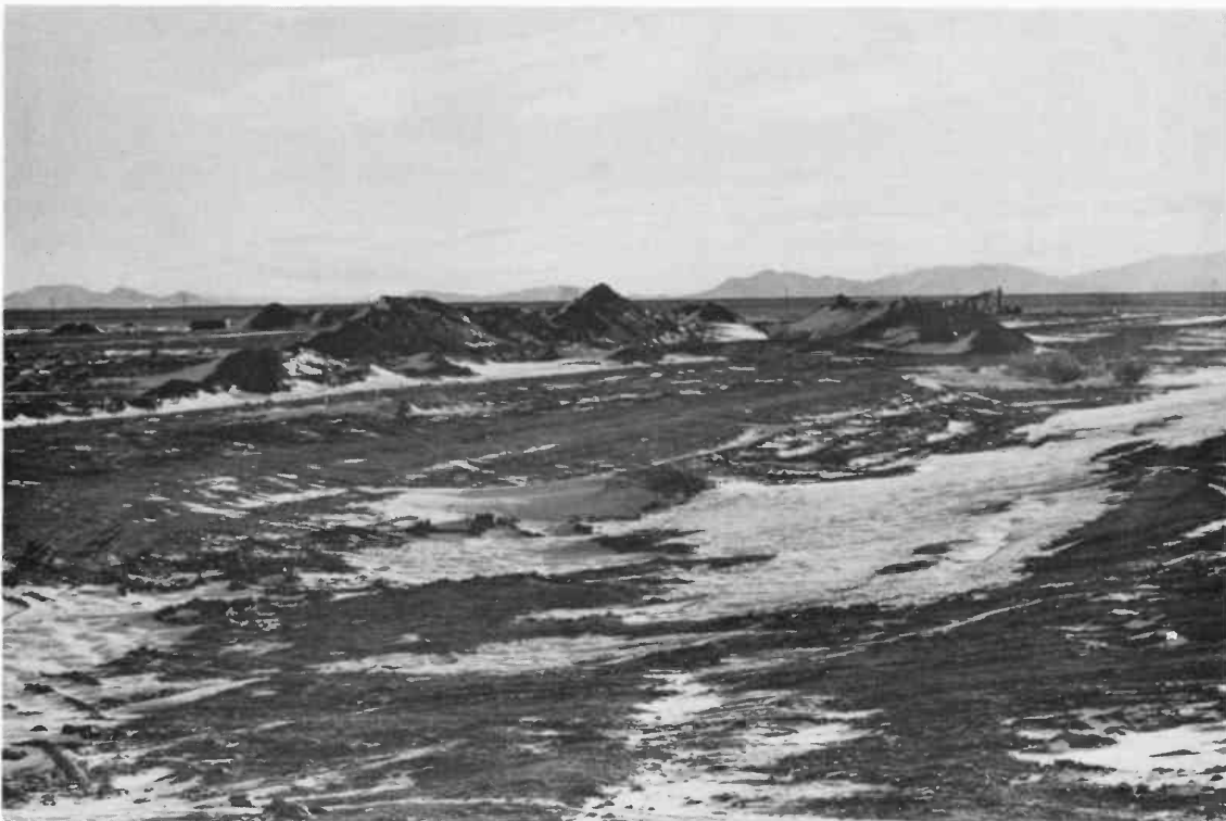
P-2. Site of Worker Housing at IPP Generating Station, December 1981
