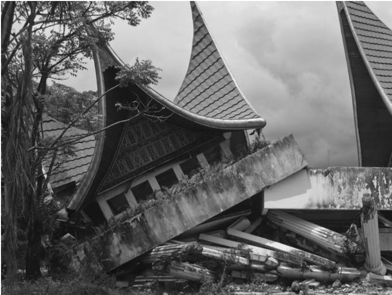
FIGURE 7.3 Aftermath of the 2009 West Sumatra earthquake in Indonesia
