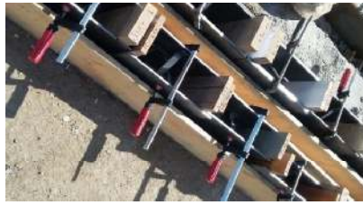
(a) Concrete molding
