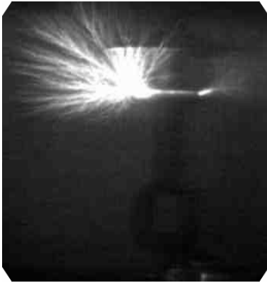
(a) Corona on hardware at 75 kV (1.1 p.u) under dry conditions
