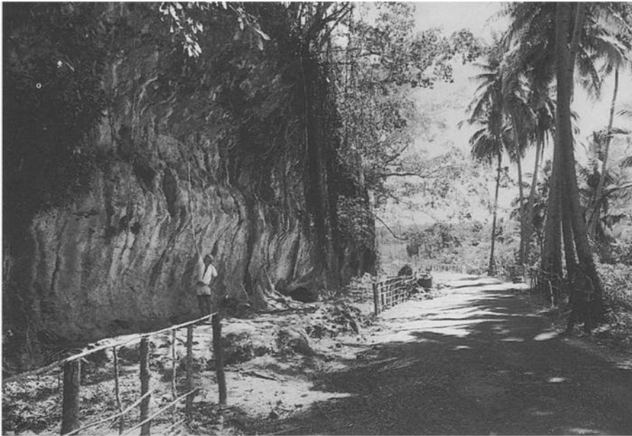
Fig. 5. Double notch at 5.0 m and 8.6 m respectively above the MLWST level near Bujanta. Scale is 2 m
