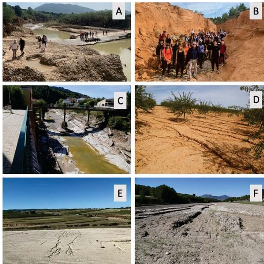
Figure 1. Views of the impact of the DANA of 12 September 2019 at the study area of river Canyoles watershed. View of the river Canyoles talweg after the flood in Granja de la Costera, (A), gully formed as a consequence of the mismanagement of the railway flows at Font de la Figuera (B), talweg of the river Canyoles in Moixent with the removal of the sediments (C), almond plantation affected by rilling in Font de la Figuera (D), rill development in sunflower fields in Moixent (E), and barley field after tillage with wide gullies in Font de la Figuera (F).
