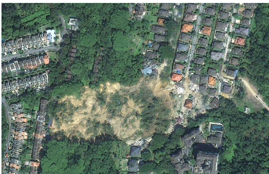
Figure 4.15: Aerial View of the Bukit Antarabangsa Landslide on 6 December 2008
