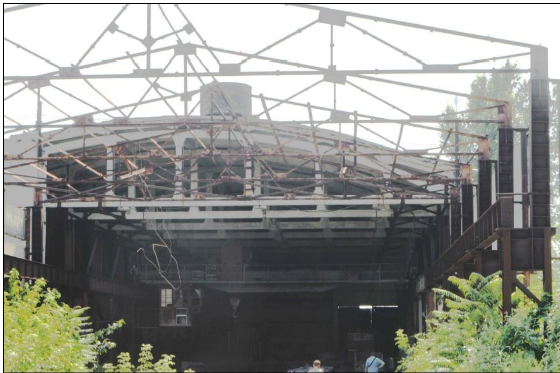
Fig. 1. Object of the research – short-span industrial storage building
