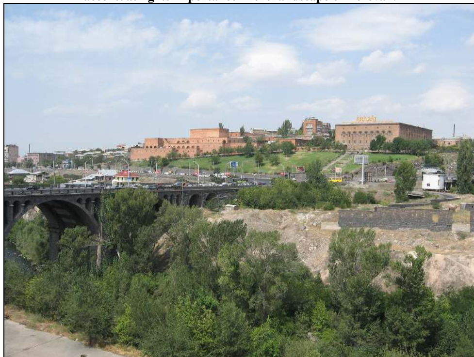
Figure 5.2: The building of the Ararat Brandy Factory in Yerevan. The word “Ararat” graces the top of the building, and a spectacular view of the mountain opens up from the factory.
