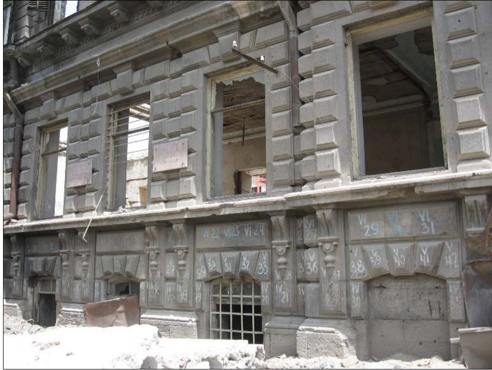
Figure 4.5: A "black building" with its façade stones numbered.
