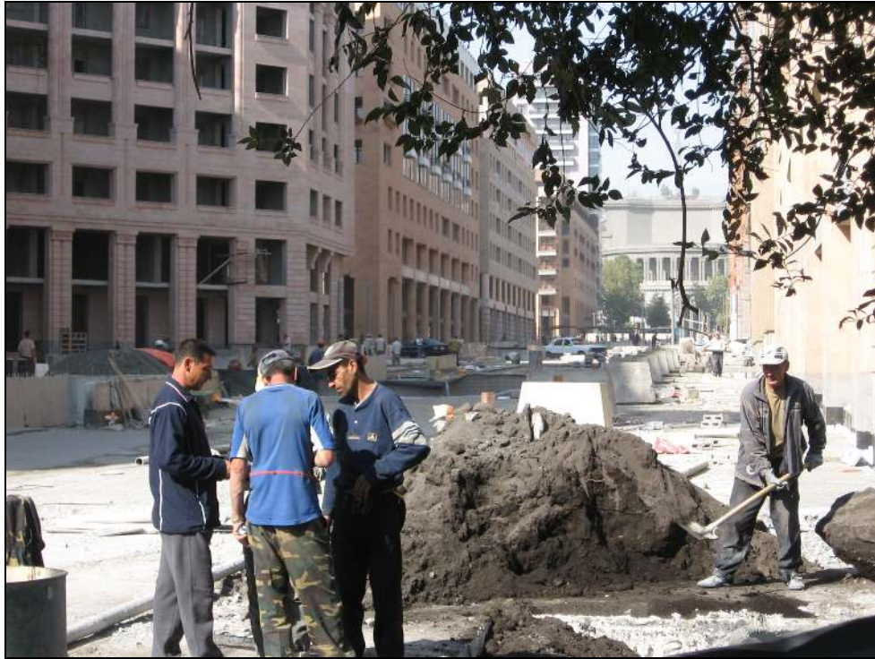
Figure 5.7: Northern Avenue, close to completion
