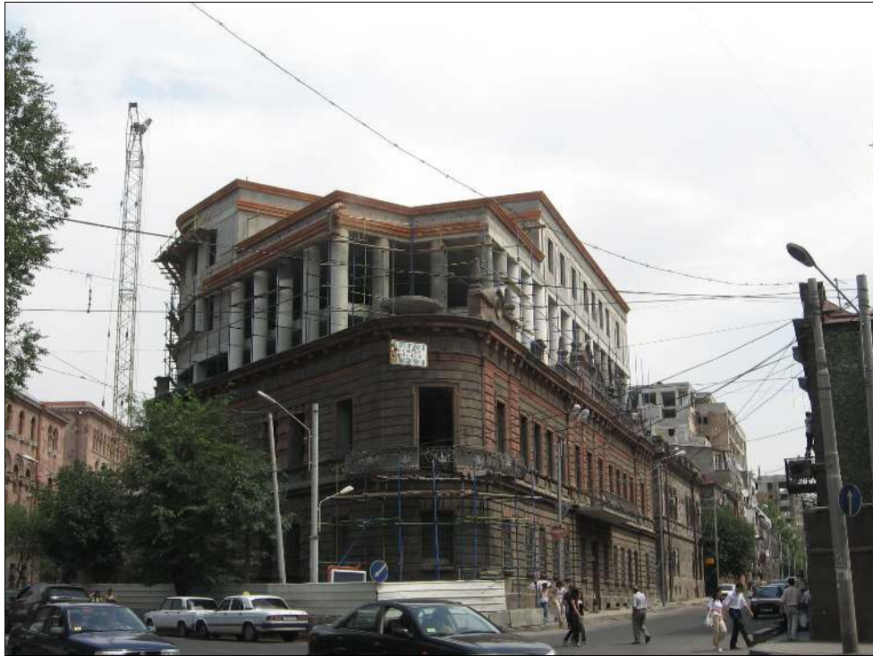
Figure 4.7: A "black building" on Hanrapetutyán Street. This building is being restored on site.
