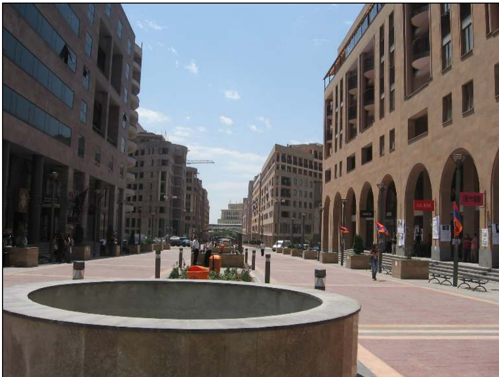
Figure 5.10: Northern Avenue in the summer of 2008. On the right side of the photo the tri-colored Armenian flags are hung where protesters of March 1st elections carried out their sitting strike. The building of the National Gallery of Arts, located on Republic Square, can be seen in perspective.
