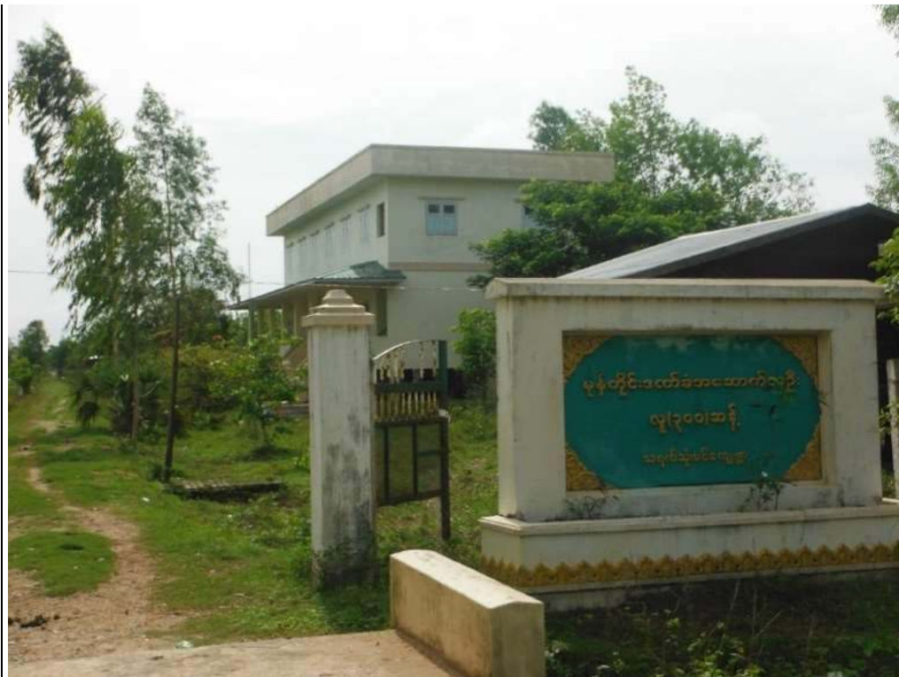
Figure 17 School-cum-shelter in Thayet Thone Bin village
