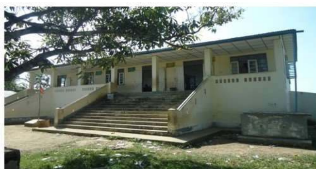
Ywar Thar Yar village school/shelter (elevated)
