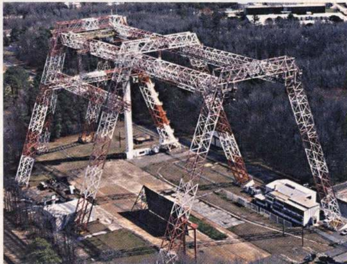
NASA Langley maintains an impact dynamics research facility, 400 ft. long and 200 ft. high, to conduct crash testing of full-scale aircraft under controlled conditions, yielding data from onboard instruments and from cameras on the plane, frame, and ground.
