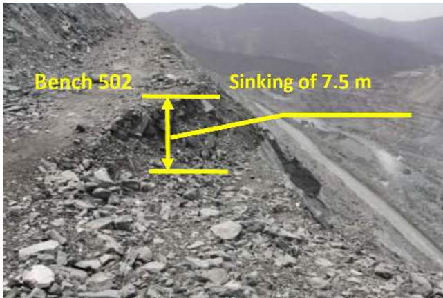
Figure 3. Sinking observed on the top of the slope.
