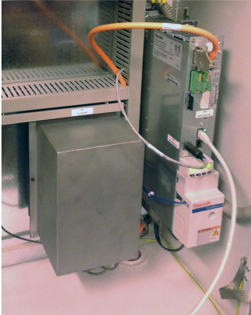
*Figure 45. Shield over frequency inverter installed*
