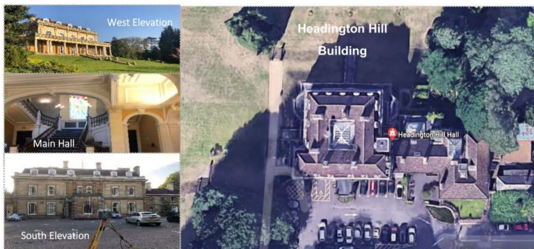
Figure 3. 3D model and aerial view of Headington Hill Building.
