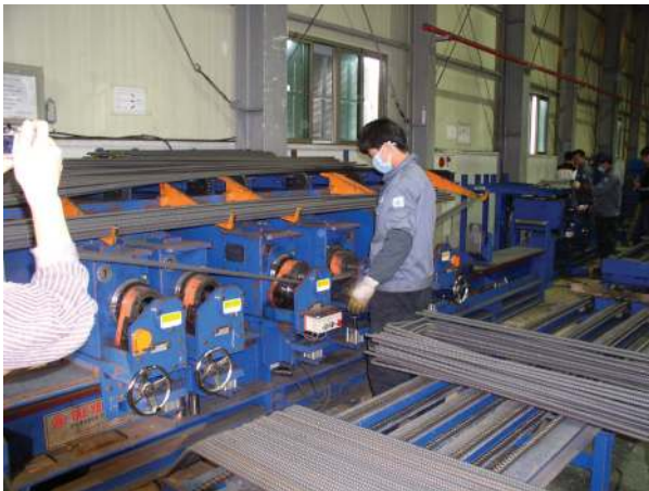
Figure 4. Field processing of rebar
