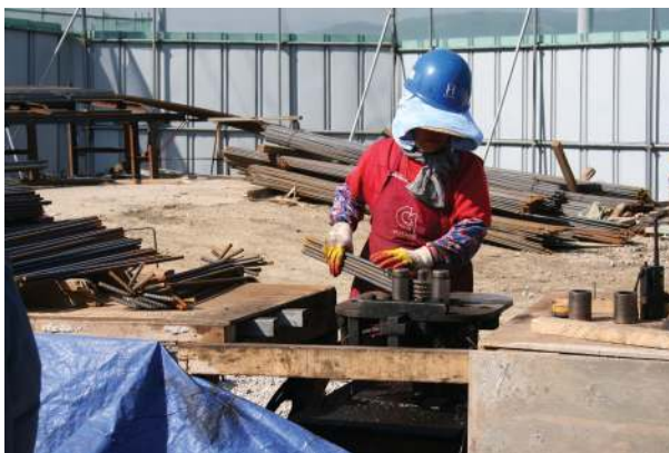
Figure 5. Factory processing of rebar
