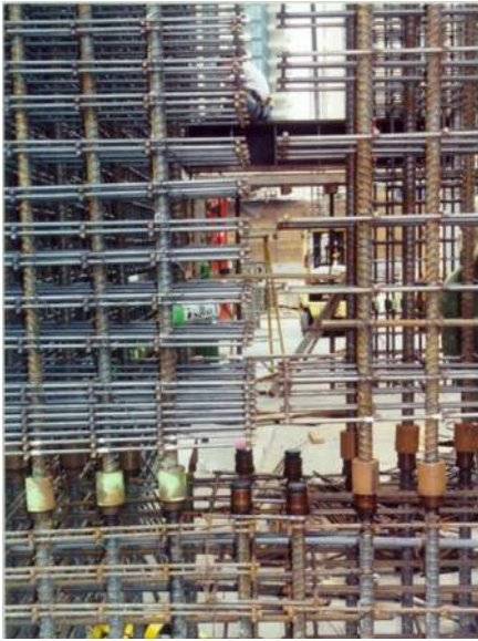
Figure 4 - Proprietary connection method allows rapid erection of elevator core cages
