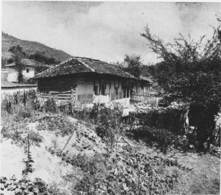
Pl. V - HOUSE IN SANGECHAL -- The large amount of timber used in the walls is an innovation after the 1957 earthquake. The roof is (as in 1957?) of wood shingle. The mound and garden in the left foreground mark the foundations of a house which was destroyed in the 1957 earthquake. 180 people out of a population of about 4000 were killed by the earthquake in Sangechal.
