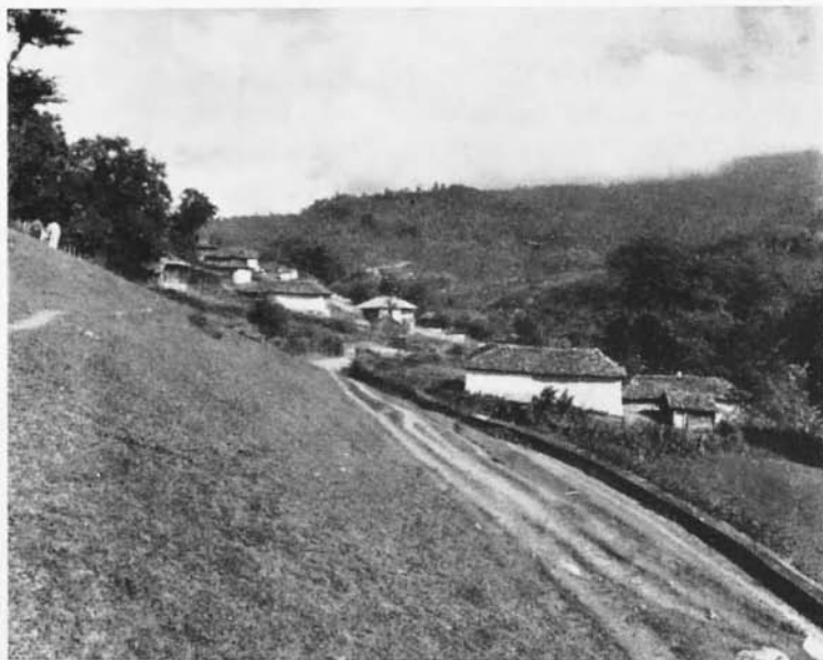
Pl. VI -- WESTERN ENTRANCE TO SANGECHAL --- The path on the right is located along one of many old landslide scarps.
