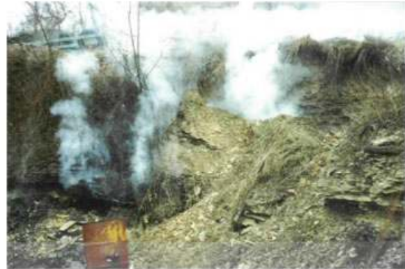
(b) Mine Fire Damage
