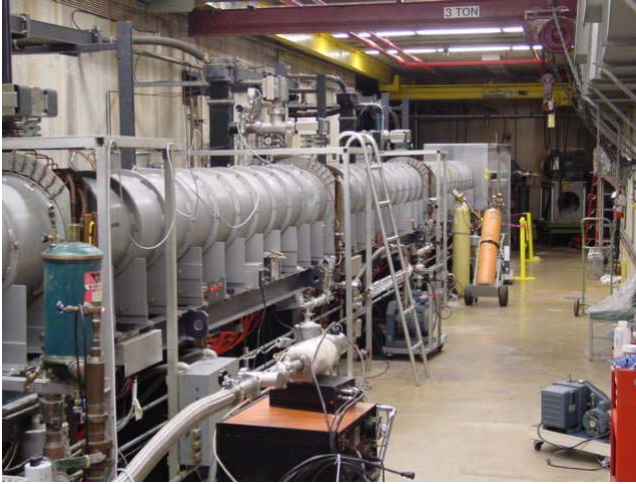
Figure 2: The ORELA Accelerator room.
