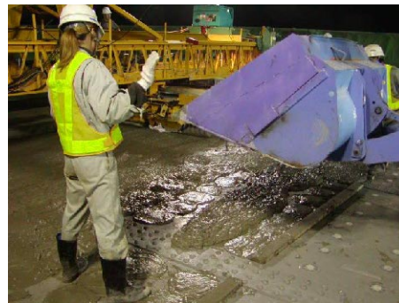
(c) Placement of HPFRCC
