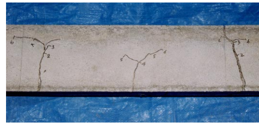
(a) Mortar specimen
