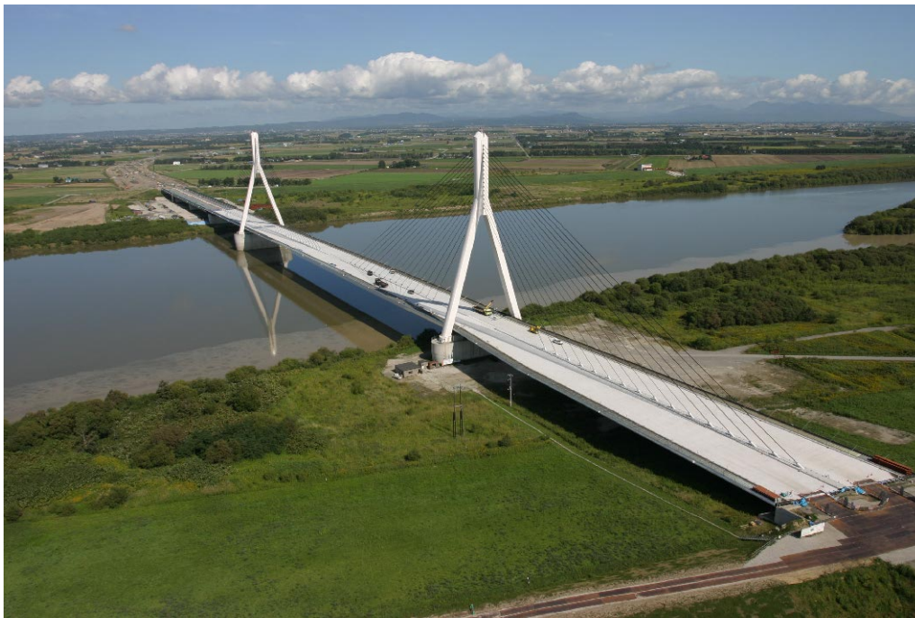
(a) Overview of bridge
