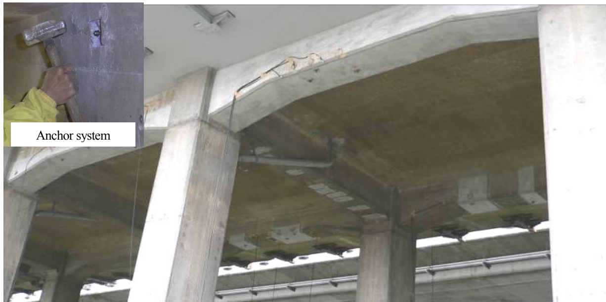
Fig. 17 Surface repair of railway viaduct.
