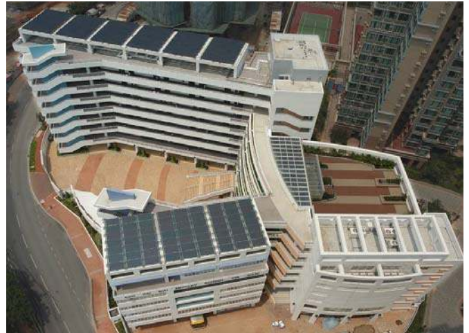
Figure 3: The completed Ma Wan Primary School with 3 BIPV
