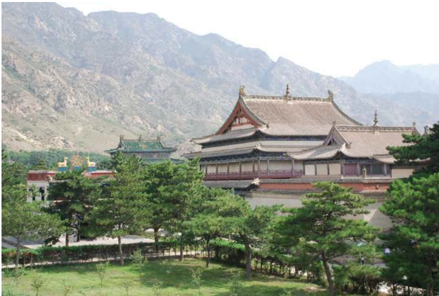
Fig. 4: Main Assembly Hall and Liulidian in the background and on the left, the small Tibetan-style Nayicung Temple
