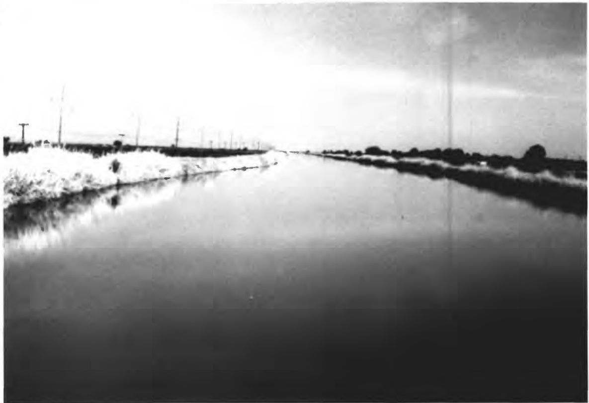
FIGURE 4. -- The All-American Canal (looking east, near Calexico).
