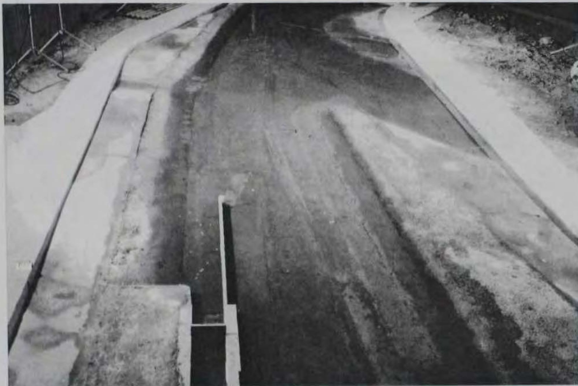
Photo 37. Plan D-2, looking downstream, showing the lower lock approach
