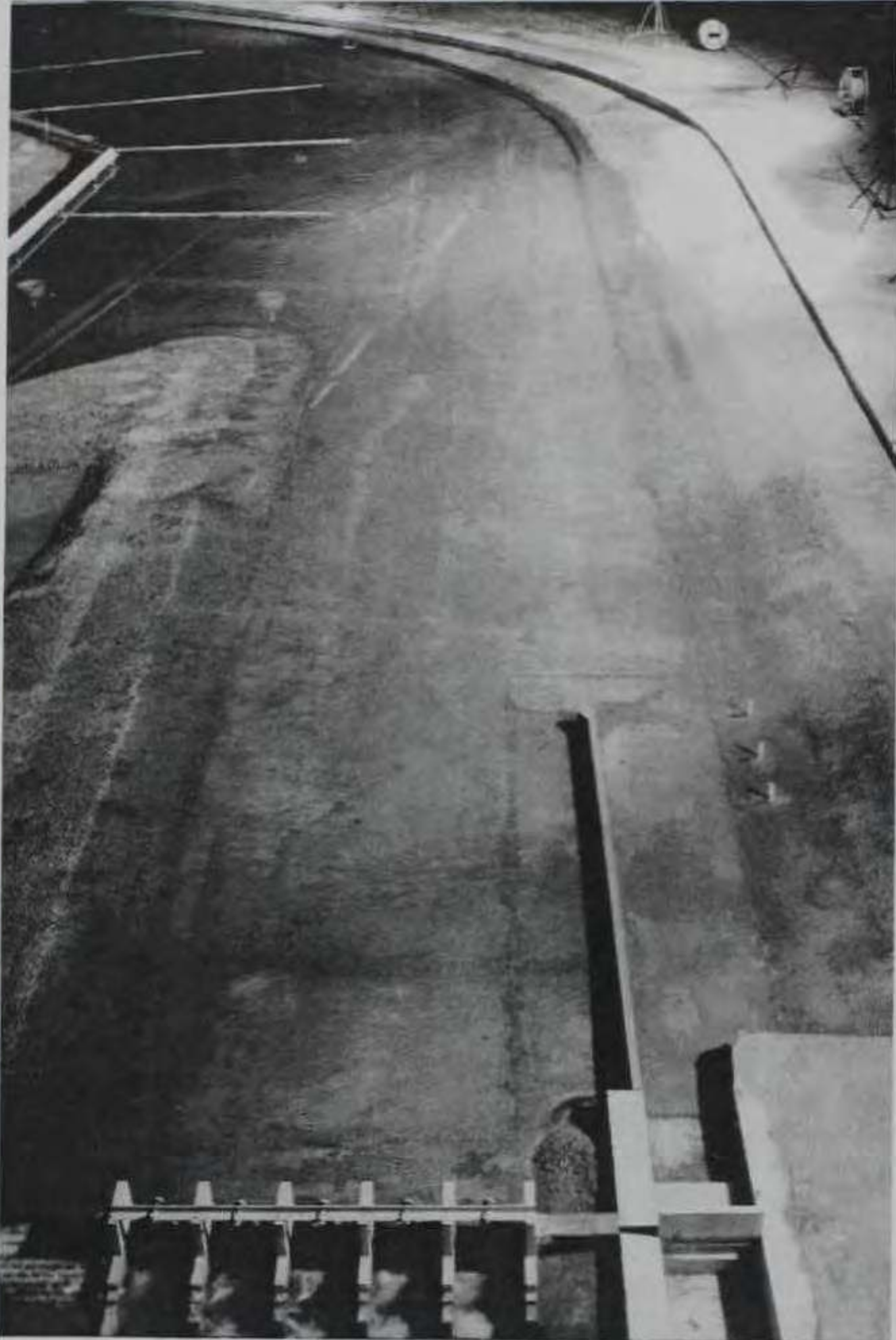
Photo 24. Plan D, looking upstream, showing the upper lock approach
