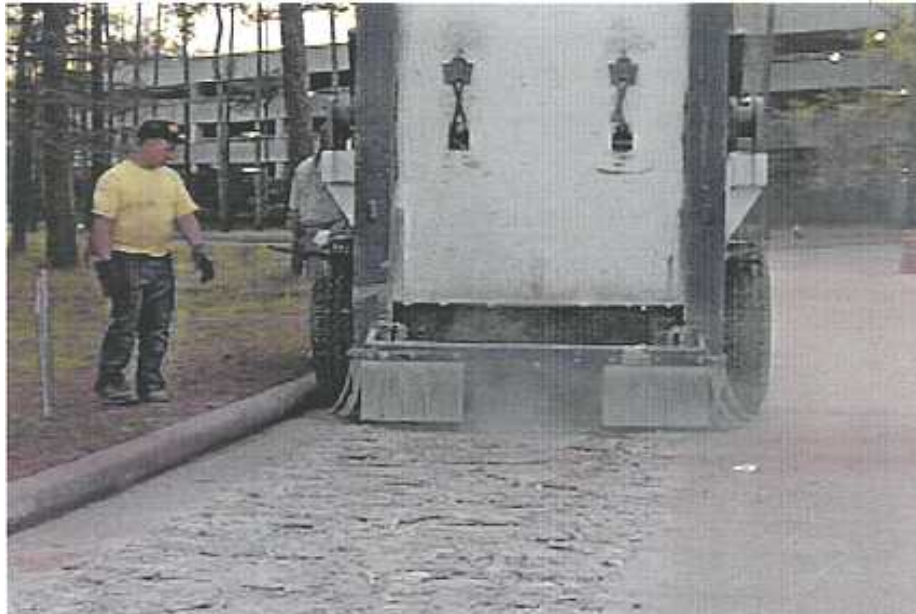
FIGURE 7 Guillotine breaker used on accelerated intersection reconstruction project.
