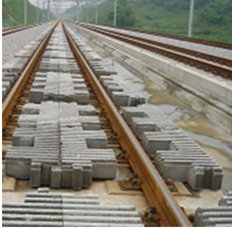
FIGURE 18: Photo of the test section.
