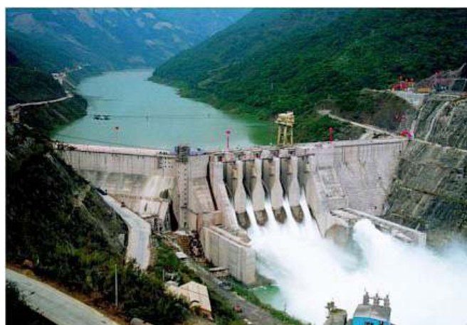
Figure 5. Dachaoshan spillway. Source: MD&A (2018).
