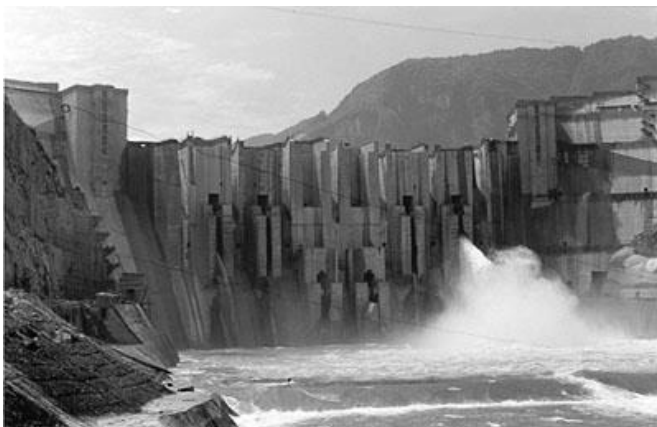
Figure 1. Slit Bucket at Geheyan Dam in China. Source: China Gezhouba Group International Engineering Co. Ltd (2010).
