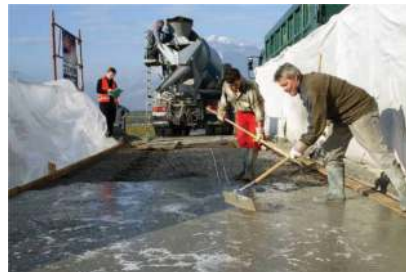
Figure 10. UHPFRC casting and handling of UHPFRC using simple tools.
