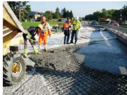
Figure 16. UHPFRC casting for R-UHPFRC strengthened zone over a pier.
