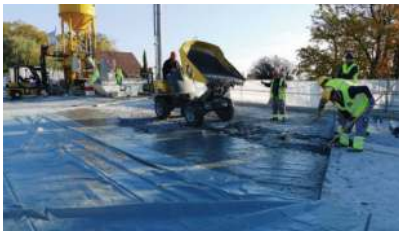
Figure 11. On-site production and casting of UHPFRC.
