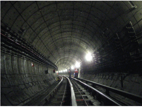
Fig. 1. Underground railway tunnel in London
