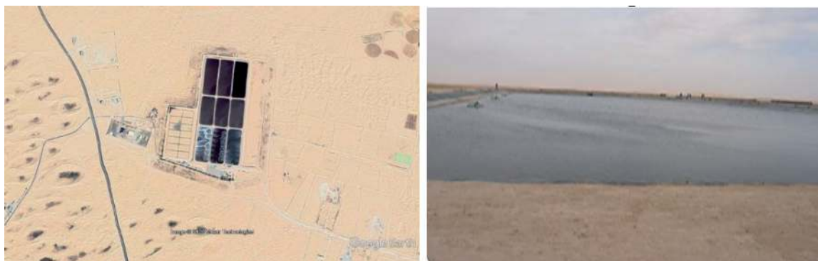
Figure 9. Kouinin wastewater treatment plant.
