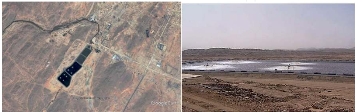
Figure 7. Tamanrasset wastewater treatment plant.
