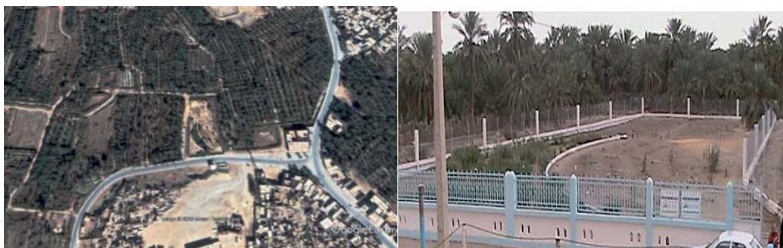
Figure 12. Temacine wastewater treatment plant.
