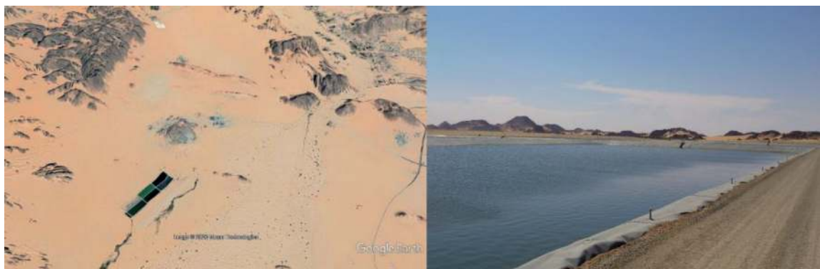
Figure 4. Djanet wastewater treatment plant.
