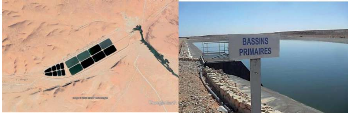
Figure 2. Ghardaia wastewater treatment plant.
