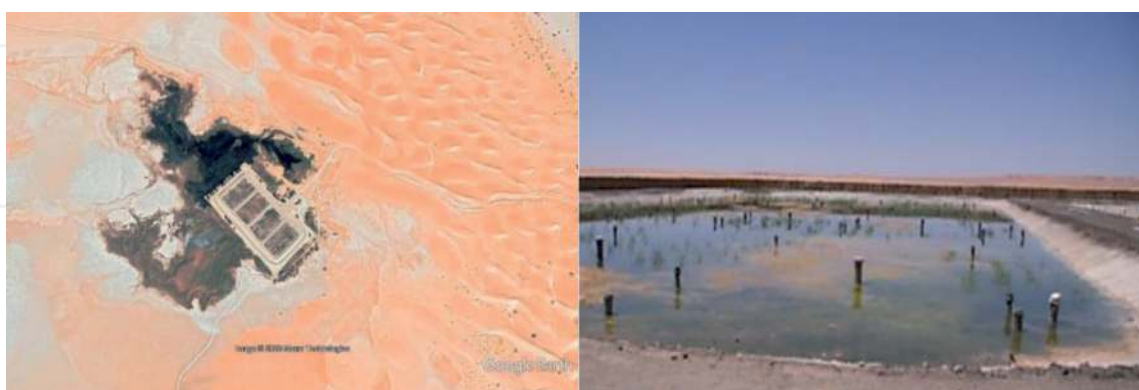
Figure 13. N'Goussa wastewater treatment plant.
