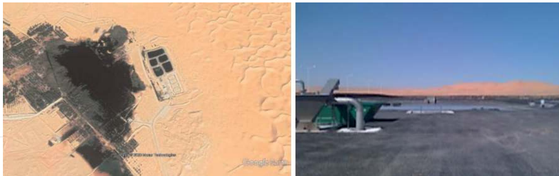
Figure 8. Sidi khouild wastewater treatment plant.
