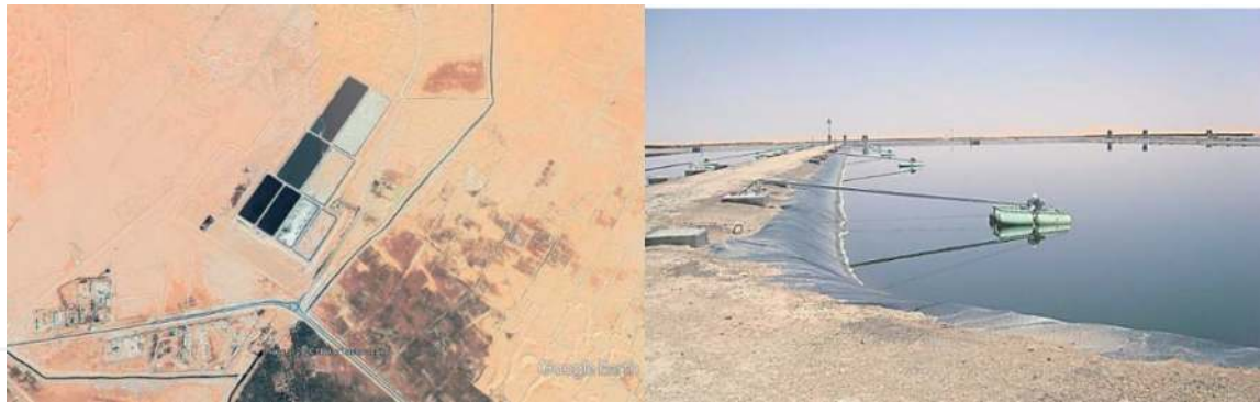
Figure 6. Ouargla wastewater treatment plant.
