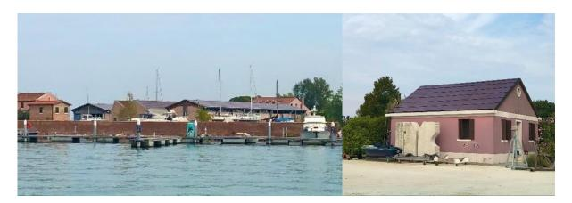
**Figure 6.** Positive example of the "*minimum intervention*" criteria on the PV roof of the La Certosa Island in Venice (Italy) with respect to the geometries, shapes, proportions, colors, and reflectance of traditional clay roofs [74] (Source: Elena Lucchi).
