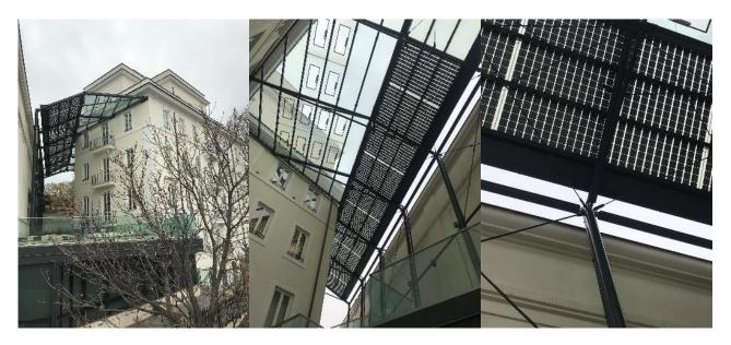
**Figure 7.** Positive example of the *"reversibility"* criteria on the solar intervention of Palazzo Leonori in Rome (Italy), where the transparent BIPV roof is detached from the original XIX Century Palace by metallic columns [75] (Source: Elena Lucchi).
