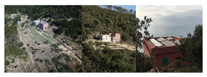
**Figure 10.** Positive example of the "concealment" of the solar intervention in the Podere Case Lovara in Levanto (Italy) thanks to the presence of traditional PV and ST panels hidden behind a parapet and not visible from the protected landscape of the Cinque Terre Natural Park (Source: Fondo per l'Ambiente Italiano).
