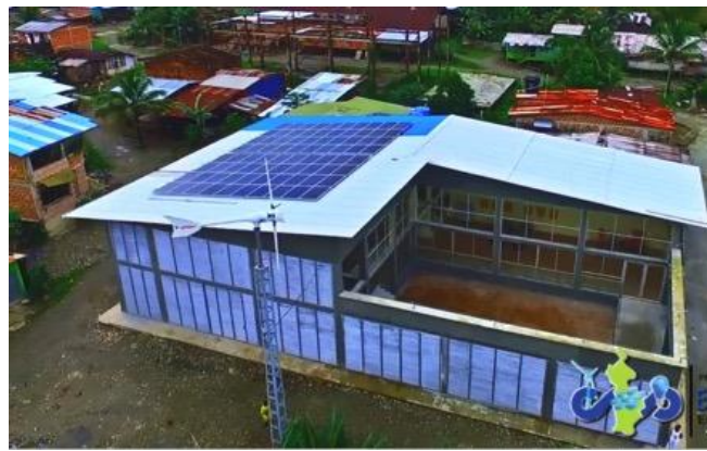
Figure 1. Photovoltaic system of 20 kW installed in Andagoya - Chocó, Colombia
