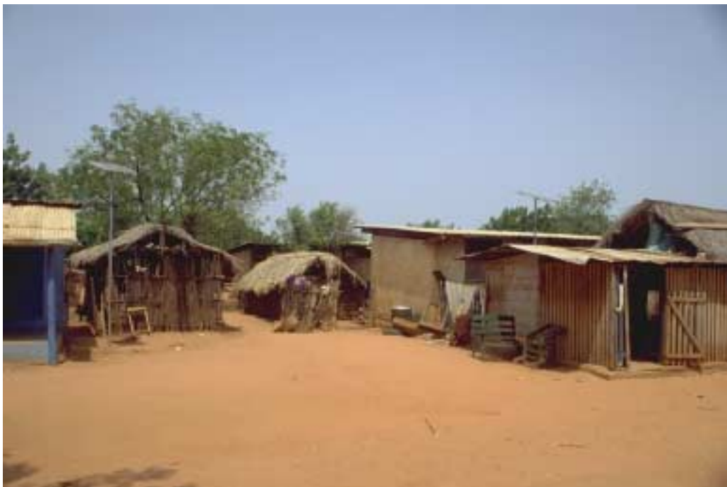
Figure 9. Rural Electrification Project in East Mamprusi District, Ghana
