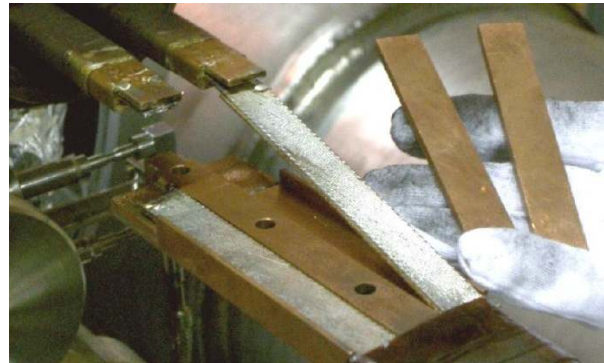
Figure K3: RQF bus-bar following the String 2 incident
