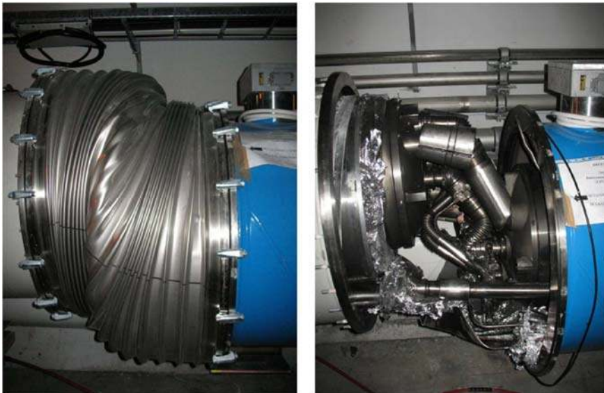
Figure 14: Damage to interconnection QQBI.27R3 by excess compression
